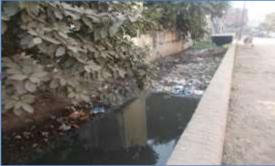
Figure 3: Katra drain with partial roofing.
